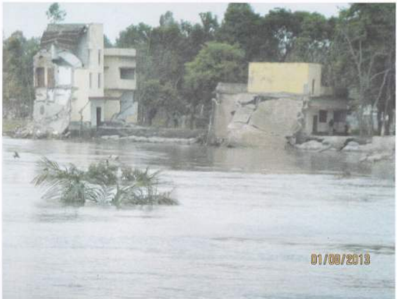
Picture-4. Showing Upazilla Parishad office buildings are going under water due to river erosion in the year-2013.
